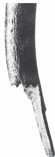
Example of corrosion failure
